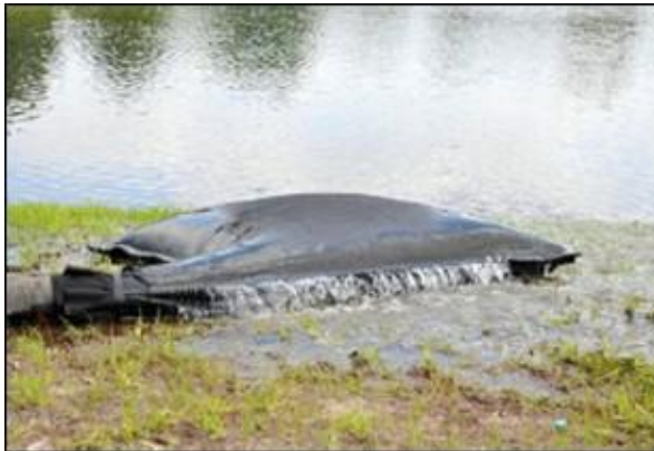
Plate 4-7 Silt Bag with water being pumped through
