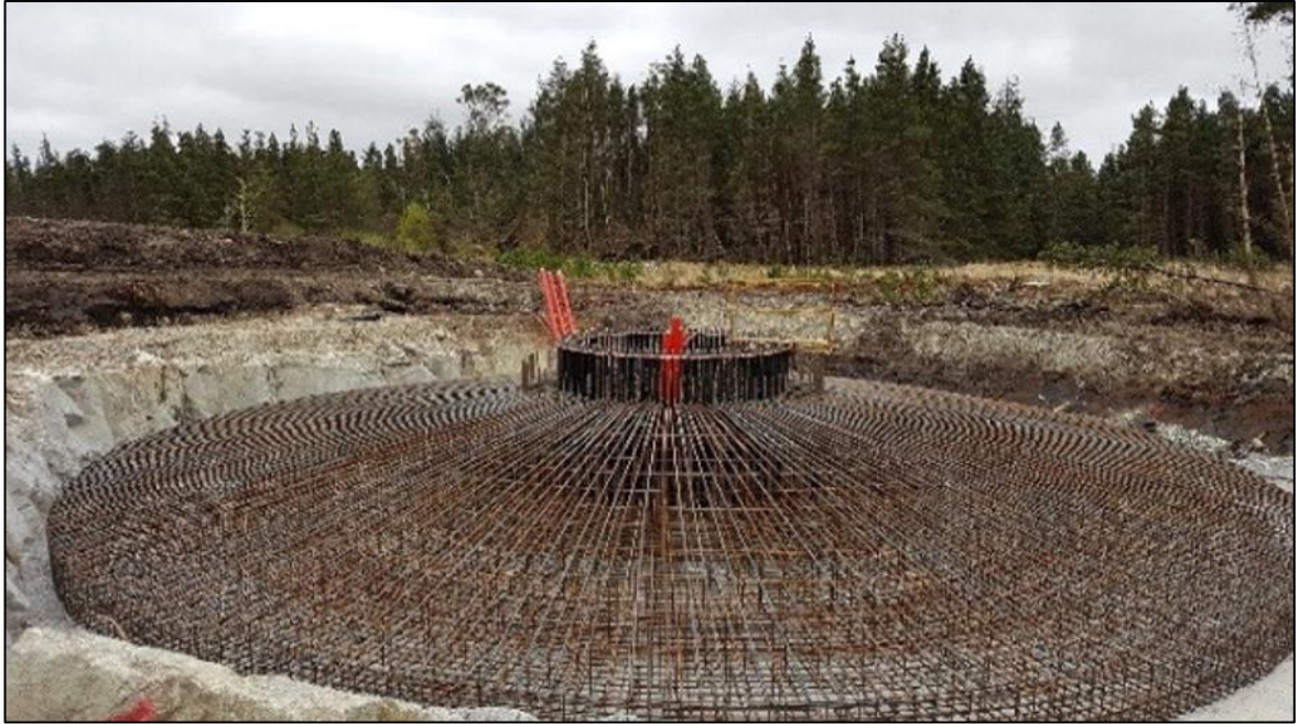
Plate 4-2 Turbine Foundation Anchor Cage surrounded by reinforcing steel.
