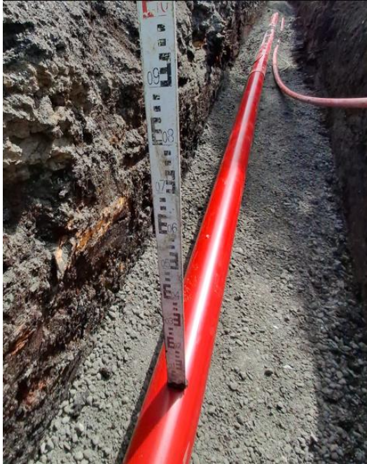
Plate 4-9 Typical Single Cable Trench View
