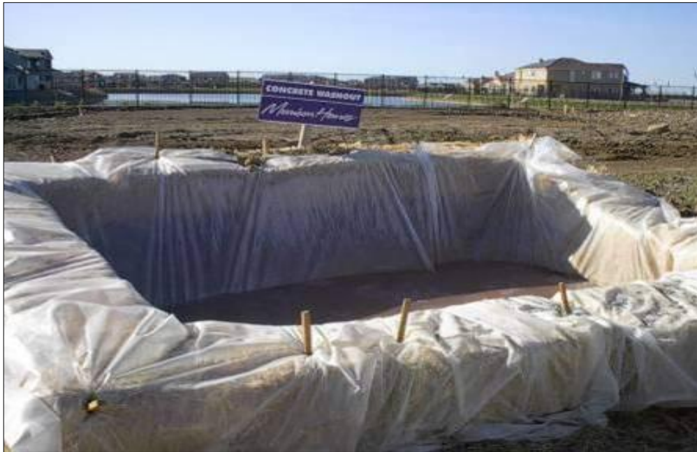
Plate 4-4 Concrete washout area
