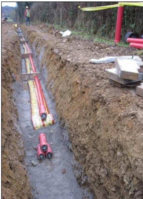
Plate 4-10 Typical Trefoil Cable Trench View
