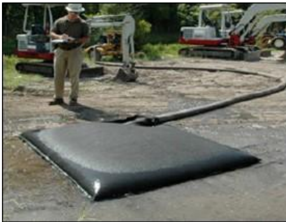
Plate 4-6 Silt Bag under inspection
