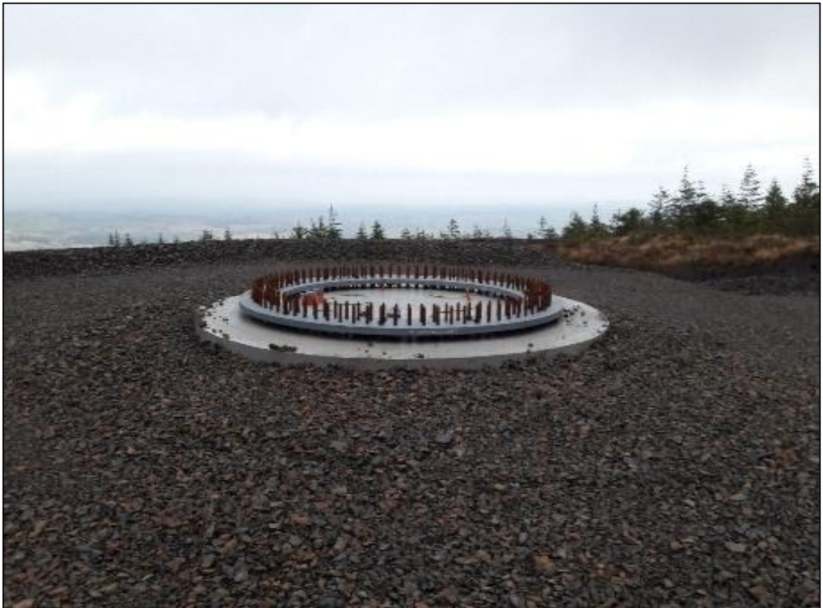
Plate 4-3 Finished Turbine Foundation
