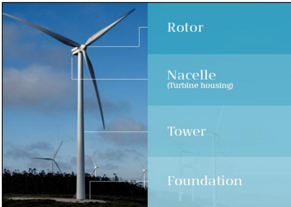
Plate 4-1 Wind turbine components
