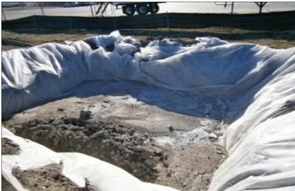
Plate 4-5 Concrete Wash Out Area
